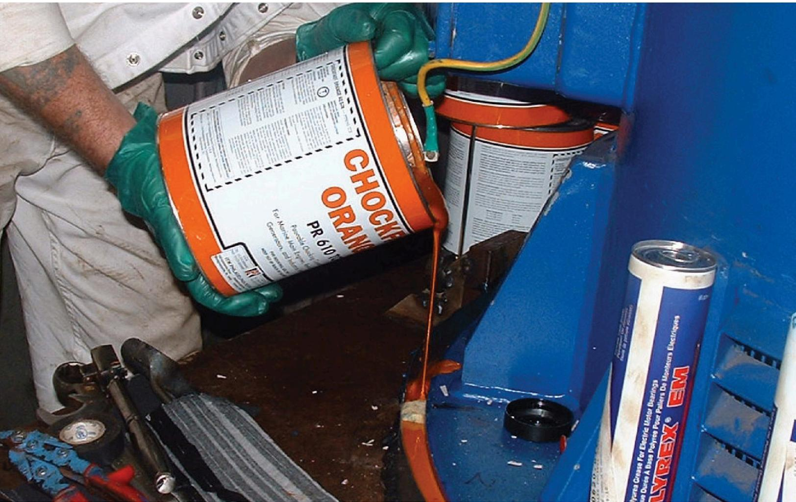
A structural epoxy “chock” or “poured shim” can replace tediously fitted steel chocks or shims.
